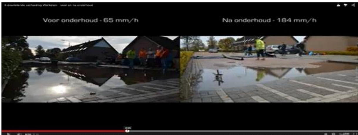
**Figure 6** visualisation by time-lapse camera showed the infiltration capacity before and after maintenance of permeable pavement at the same time on video (<http://www.climatescan.nl/page?details=60>). (Tipping, 2015)
