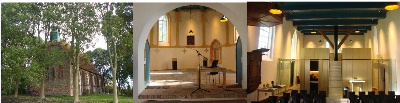
Figure 2: Leegkerk a) exterior; b) apse with storage doors; c) nave with glass draught lobbies. [18]
